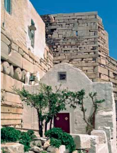
119. Section of the walls of Paroikia castle; Agia Anna's chapel.
