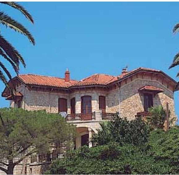
99. A mansion in Poseidonia, housing the Town Hall.
