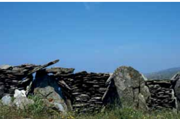
66. Traditional dry stone wall in a rural area.
